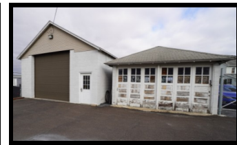
Garage / Work shop
