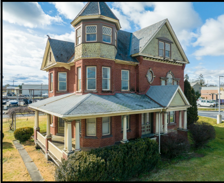
Above: Victorian Building
